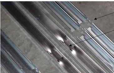
Please note that 2 of the tracks have a pass-through hole and 2 tracks that have a swag (impression) in the center.
