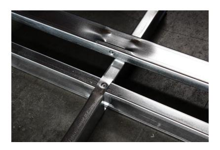
Push the stud with the swag threw through the track with the holes punched in them. Align the dimples and place a screw in the joint.
