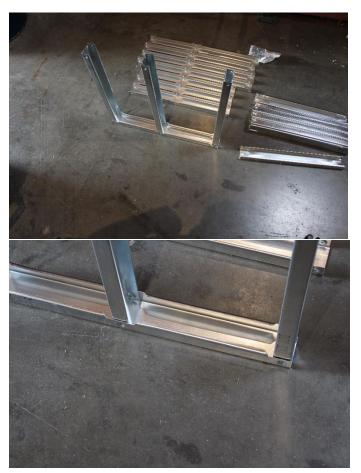
Do this for all the tracks and studs. Each section will have 2 tracks and 3 studs in them.
